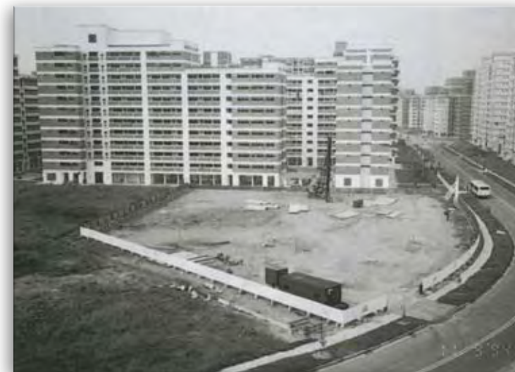
Construction of Choa Chu Kang Bible Centre, 1994
