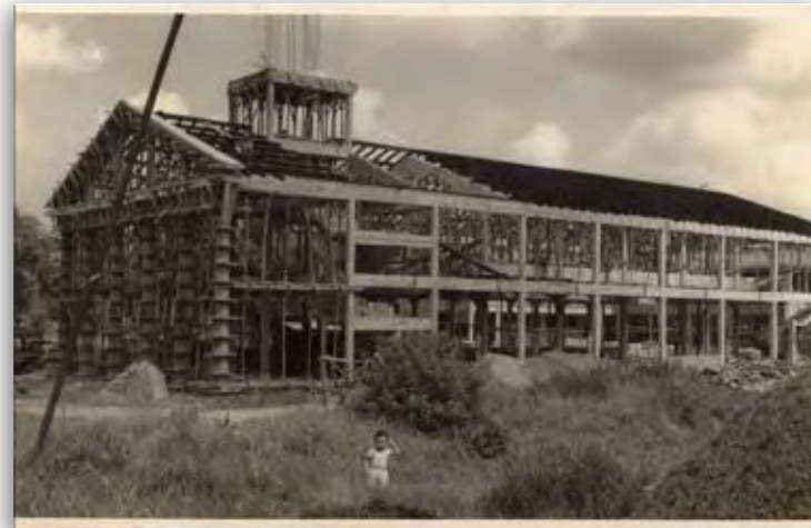
Life BPC building site, 1962
