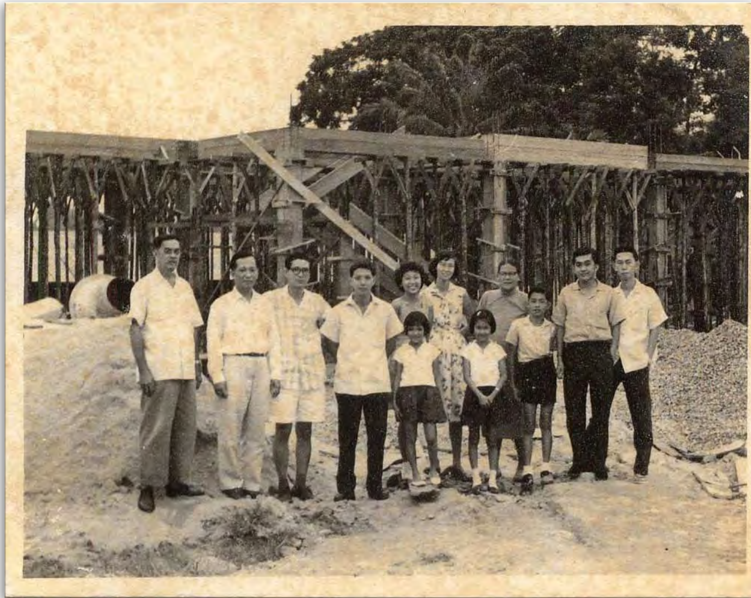
Life BPC building site, 1962
